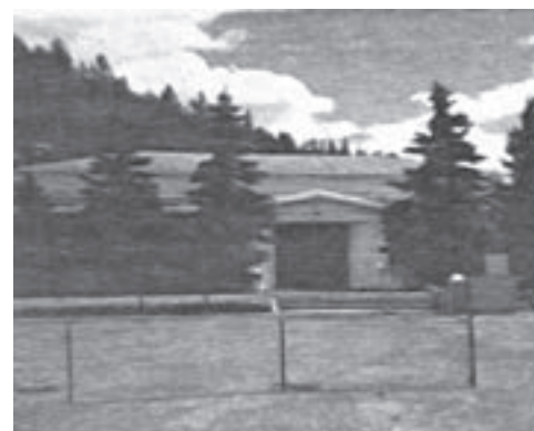
Abandoned masonry school, housed EHS and MOLS
